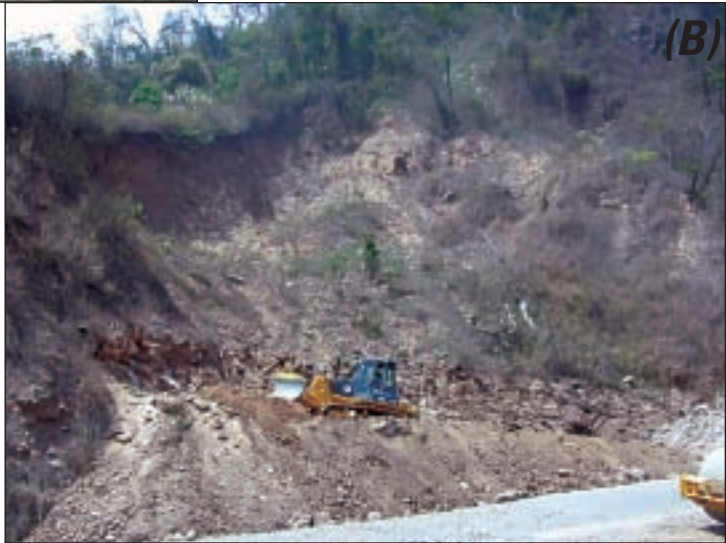
Figure 6. Landslides along the road to Jinotega in the La Fundadora study area showing broad scale of response. (A) A failure less than 1 m deep and about 40 m 2 in area. Material from the failure traveled approximately 20 m over an open hillslope. (B) An approximately 5-m-deep failure into weathered material. This landslide was approximately 3000 m 2 in area and traveled at least 100 m down a channel.
