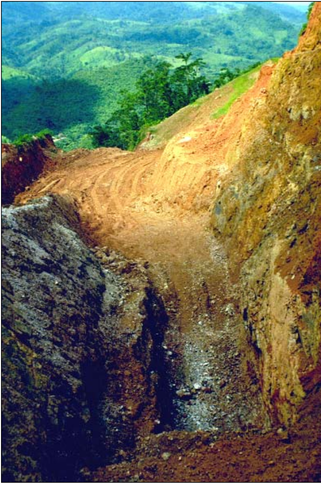
Open cut excavation of the Atlas vein at HemcoNic's mine site.
