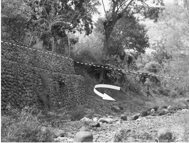
Fig. 4 Image of the concave margin of a meander. Undermining is evident below the roots of the tree, where unconsolidated sediment is being eroded ( white arrow ). The dike, built after the Mitch hurricane event, is obviously too short and undermining is beginning to act behind it and therefore it will be ripped off. The lower terrace level is indicated with a white discontinuous line . La Trinidad, 2004
