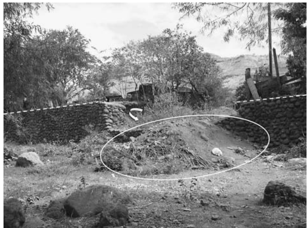
Fig. 5 Image of a filling on La Trinidad river bed indicated with a white circle . The dike, built after the Mitch hurricane event, presents a discontinuity and erosion is beginning to act behind it ( white arrow ). The lower terrace level is indicated with a white discontinuous line . La Trinidad, 2004
