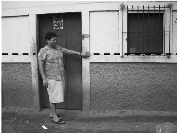
Fig. 2 Woman showing the level reached by the water during the Mitch hurricane event (black discontinuous line). La Trinidad, 2004
