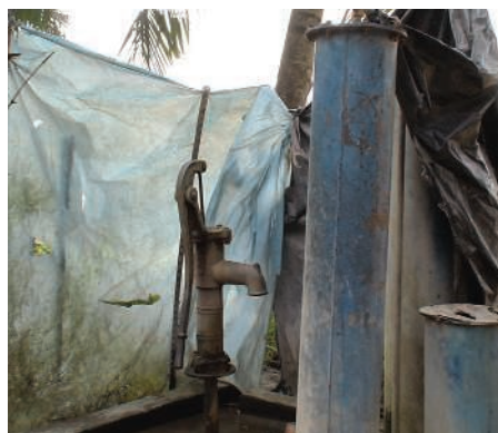
Defunct. Numerous arsenic-removal units installed by the West Bengal government no longer work due to lack of maintenance.
